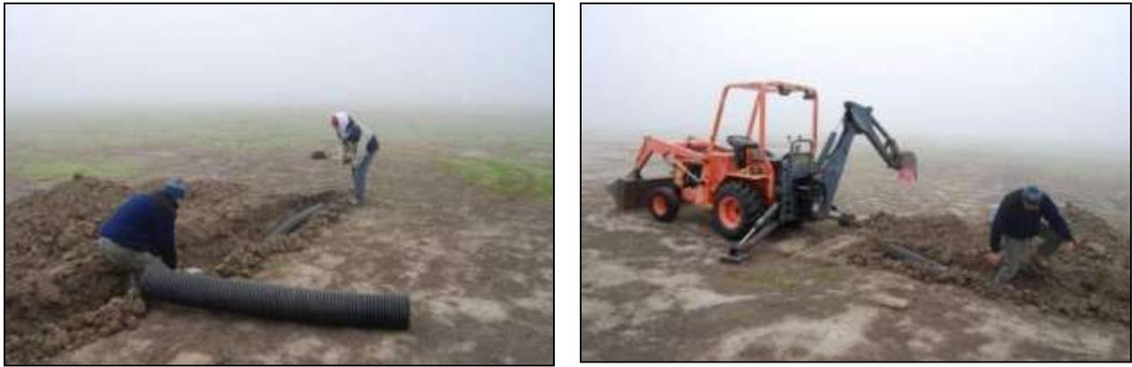
Figure 10. Installation of chambered dens in the Semitropic Ecological Reserve area, Kern County, CA.
