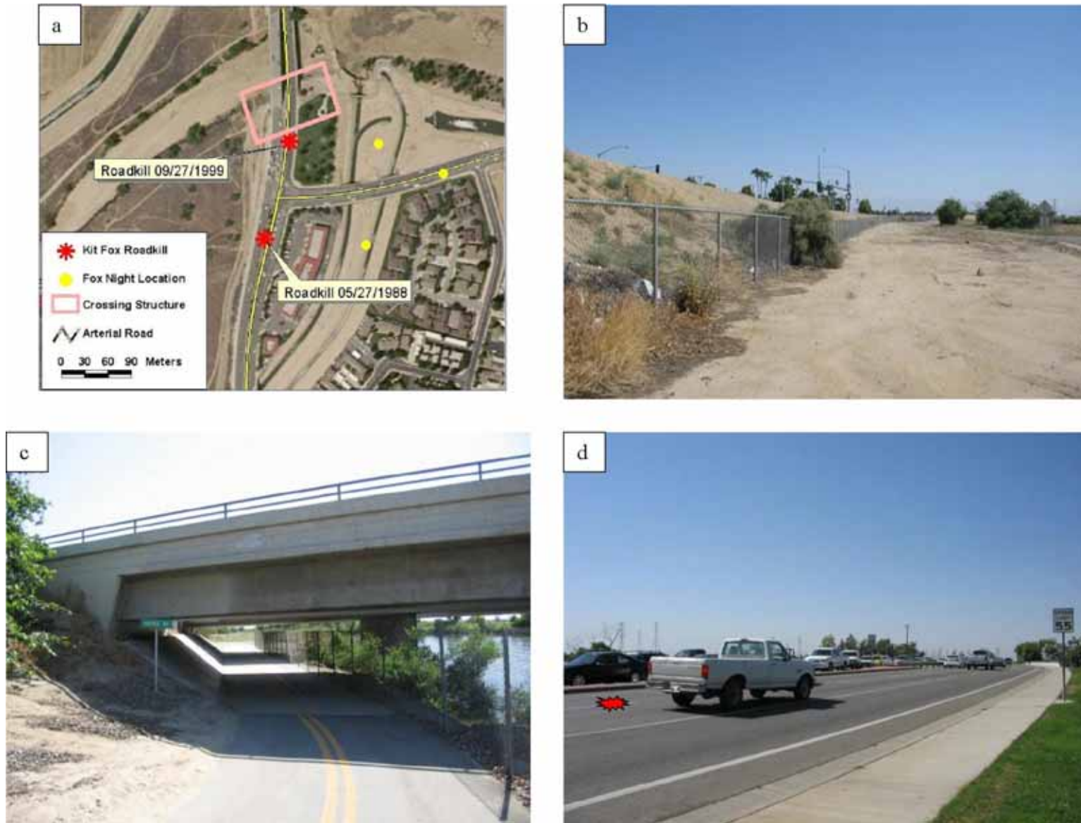
Figure 24. Coffee Road overpass at Kern River bicycle trail, Bakersfield, CA. a) Aerial view of kit fox roadkill and radio-tagged night locations at crossing structure. b) Habitat view from west entrance. c) East entrance to bicycle path on southern embankment of Kern River. d) View of roadway from East with location of kit fox roadkill in red. No fences prevent fox access to roadway on eastern side.
