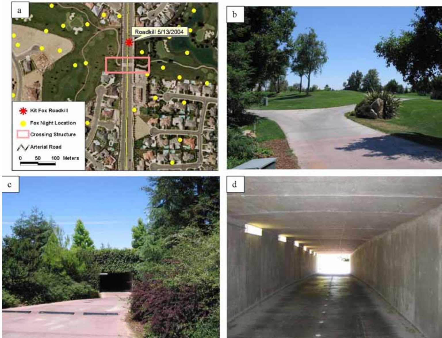
Figure 22. Buena Vista Road golf cart crossing structure, Bakersfield, CA. a) Aerial view of roadkill and radio-tagged kit fox locations at crossing structure. b) Habitat view from east entrance of crossing structure. c) Approach view to east entrance. d) Passage interior.
