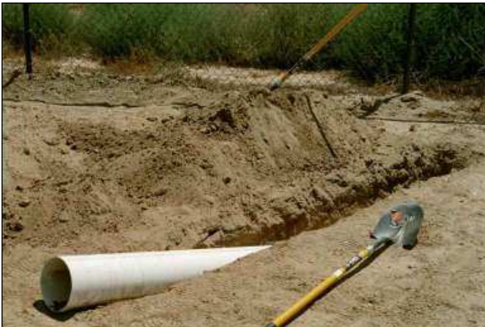
Figure 20. Installation of artificial single-entrance escape den.
