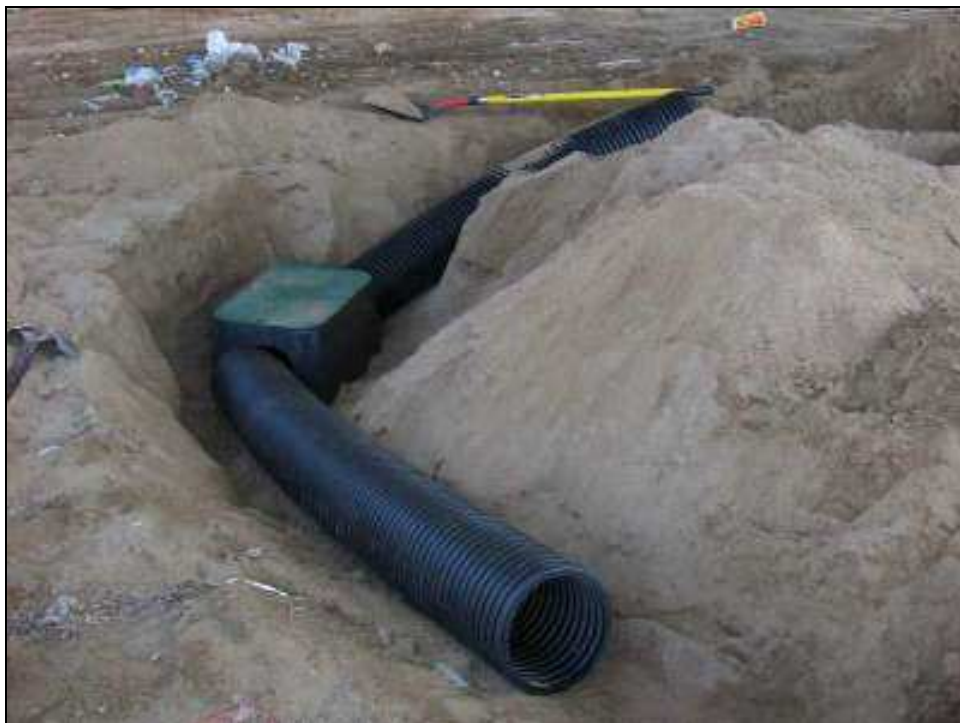
Figure 17. Installation of a residency den under school athletic field bleachers.
