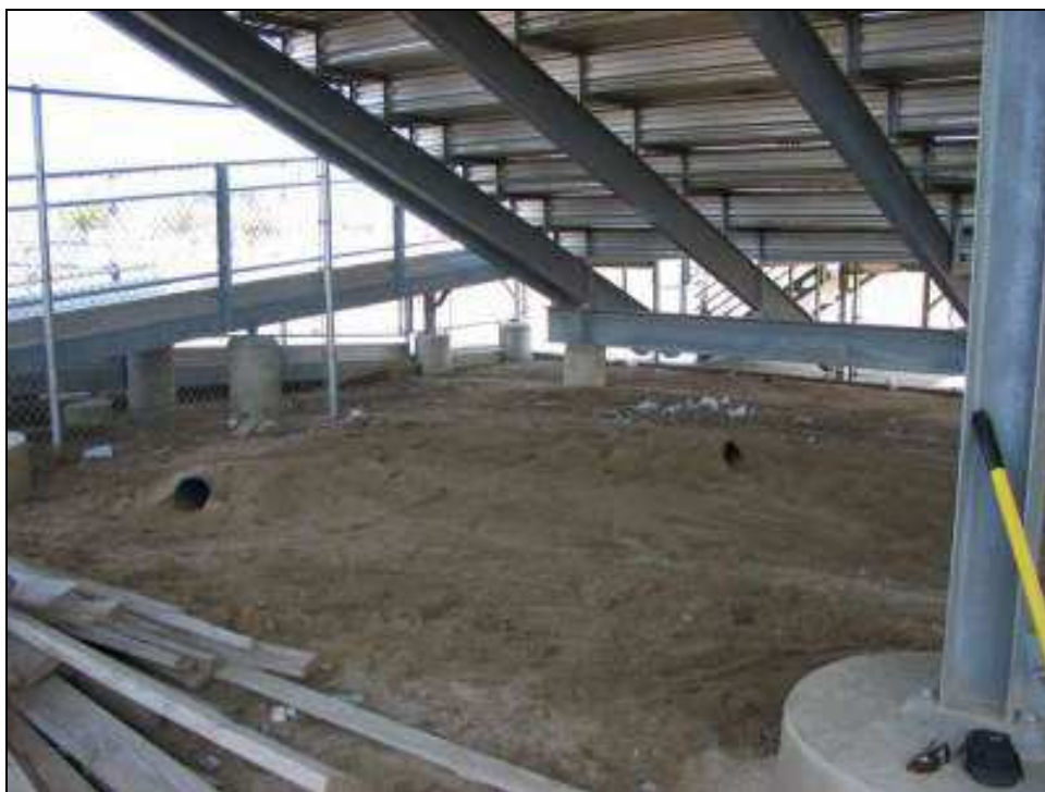
Figure 18. Post-installation view of residency den under school athletic bleachers.
