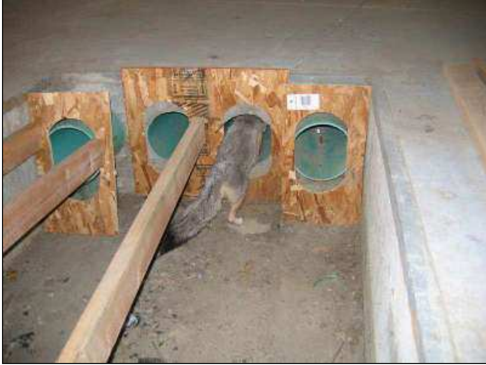
Figure 8. Kit foxes can den in below-ground infrastructure such as pipes or culverts.
