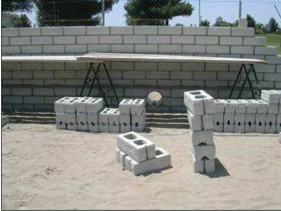
Figure 27. Wall designed with opening (b) to allow kit foxes to pass through.
